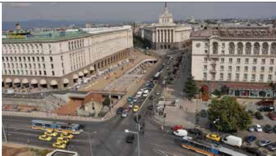
Photo 1: The largo complex, Central Department store (left)
